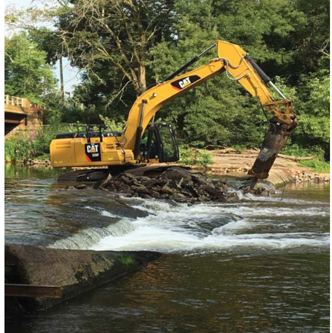
Weston Mills Dam Removal
