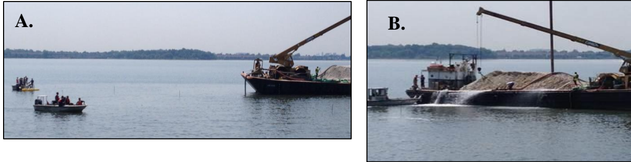
Fig. 7. A., Shell barge approaching restoration site with various partners in boats observing. B., barge deploying with pressure hose seasoned mollusc shell to construct shell base.
