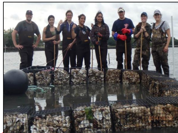
Figure 6. Gabion Blocks secured together forming a 10 ft 2 perimeter ‘reef’.
