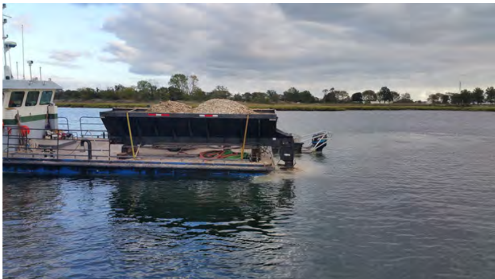
Figure 4.7 Picture of placement materials by the spreader.
