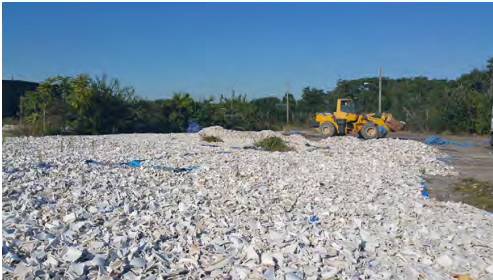
Figure 4.6 Porcelain Material "curing" prior to placement
