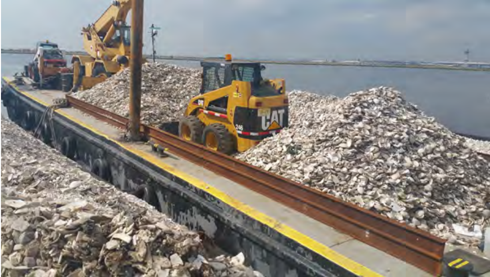
Figure 4.5 Receiver reef materials: seasoned clam shells, oyster shells and crushed porcelain
