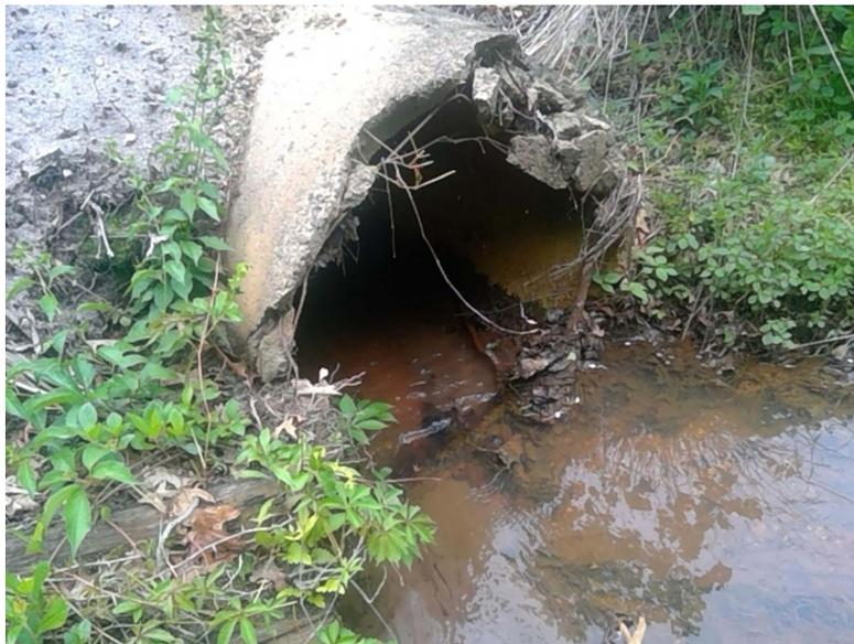
2. South River tributary A1 (SRA1) is a small culvert on an ephemeral tributary. It would not generally score very high, except at the time of assessment the inlet was completely buried in mud, debris and water, making it a high risk for roadway flooding. This crossing is in need of maintenance. The photo on the right shows the clogged outlet
