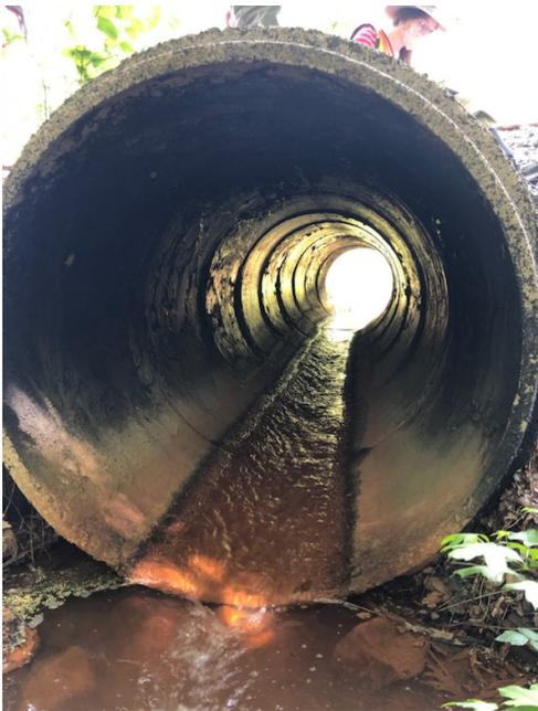
3. Selovers Brook 2 (SB2) is the most important barrier to remove for anadromous and potadromous fish in this subwatershed. The water at this railroad crossing is deep at both the inlet and outlet, and very shallow inside the culvert, indicating probable erosional issues. Improving this barrier would open up 1.2 miles of upstream aquatic habitat with full downstream access to the ocean.
