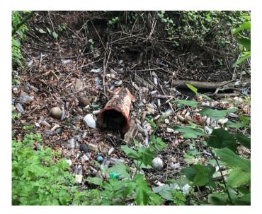
4. Long Neck 5 (@ trail behind Midland Park) is a small culvert under a paved path just upstream of the railroad crossing. This crossing is in poor condition and has been severely blocked by debris which has led to an inlet drop affecting aquatic connectivity. Maintenance is needed.
