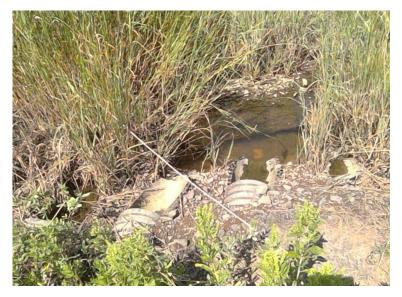
2. GD1 (@ Lorrain Ave) is the first barrier on a tributary that runs into Cheesequake Marsh from the west. This crossing is severely undersized and can only accommodate a 25-year storm event. There is also a drop and large pool at the inlet of this structure that likely ends most passage upstream at this first barrier for anadromous fish.
