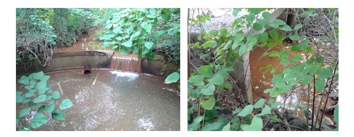
3. Long Neck 4 (@ railroad) was not able to be assessed because it is fully blocked by debris to the extent that we could not find the crossing structure. It is possible that this structure is in good condition and adequately sized but as of now, aquatic connectivity is non-existent and intensive maintenance is needed as well as an evaluation of the causes of such a severe blockage.
