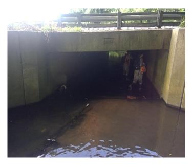
3. Mill Brook Tributary A4 (@ Hwy. 1) is a small culvert on a small tributary of Mill Brook. It has a large outlet drop that is a full barrier for aquatic passage for both anadromous and potadromous fish.
