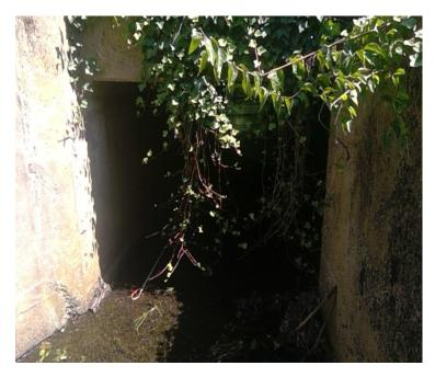
5. Mill Brook Tributary D14 (@ Orchard Ave.) is a small bridge furher up in the watershed. It is fine for fish passage but is severely undersized and is falling apart.
