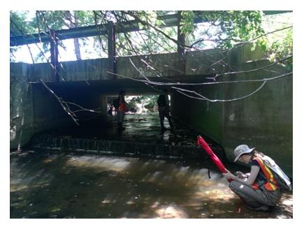
2. Mill Brook Tributary D11 (@ Rt. 1 exit ramp) is an undersized bridge that has a concrete bottom where the streambed has eroded on both the inlet and outlet sides, thus the crossing is slightly perched, has a slight outlet drop, and large pools at both the inlet and outlet side. This erosion may be due to the undersized nature of the structure. All of these factors contribute to less likelihood of fish passage for potadromous fish.
